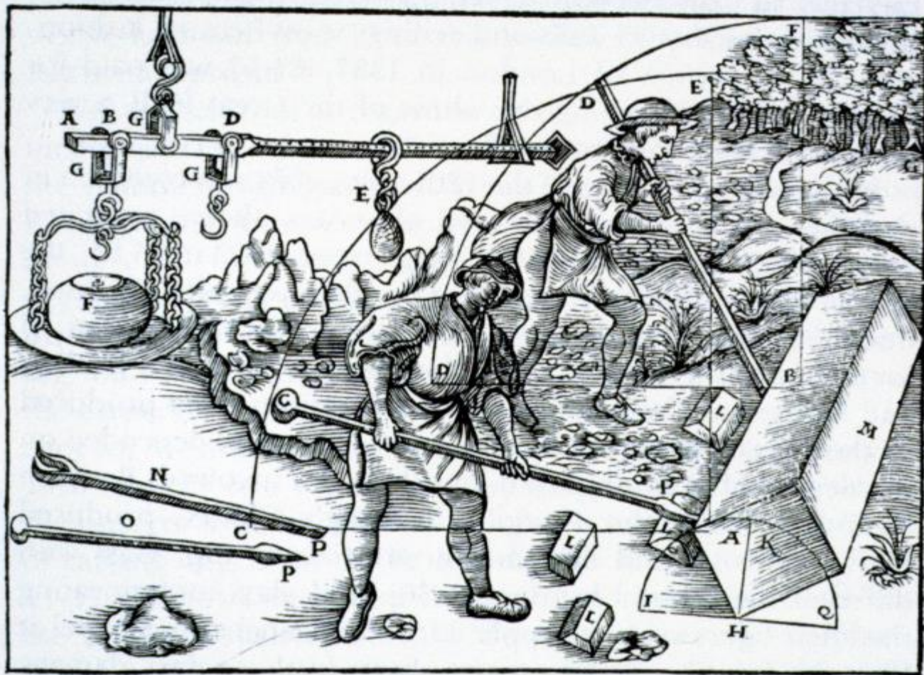
Fig. 110. Moving a pillar
